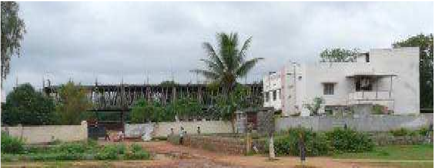
Hyderabad , above, the new building going up near the old building. Johanne Toutant photo
