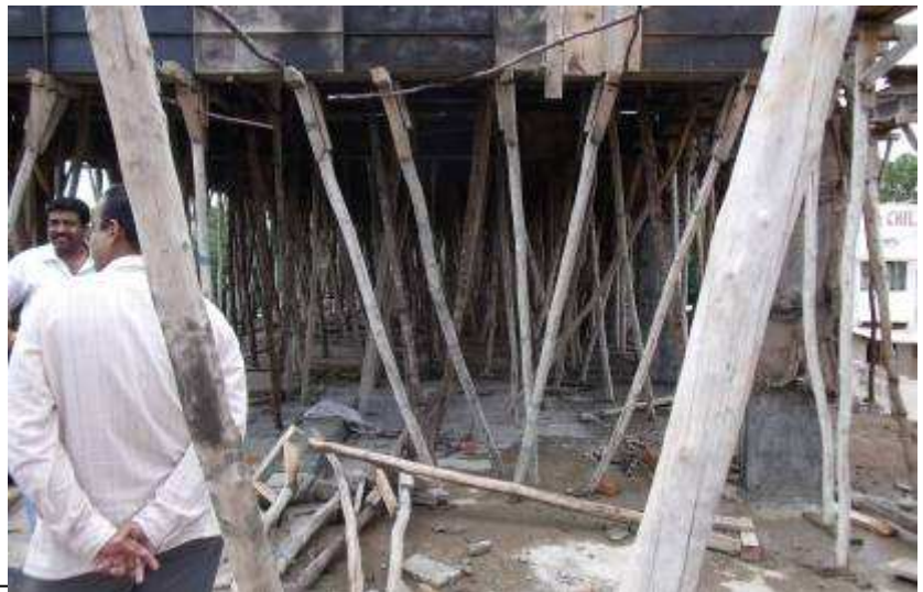
HYDERABAD , left, Intern Johanne Toutant. Above, the upper floor concrete is drying on a system of “trees”. Deverell photo
